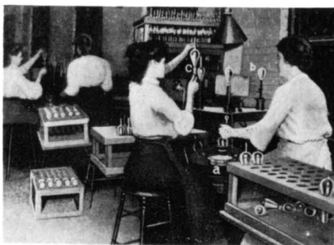
Left: Sealing machine at Westinghouse in 1910. Above: The sealing-in process as performed at Westinghouse in 1910.
